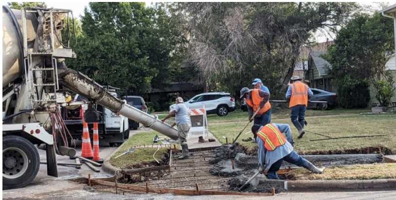
Installing ADA ramp on Harrington
